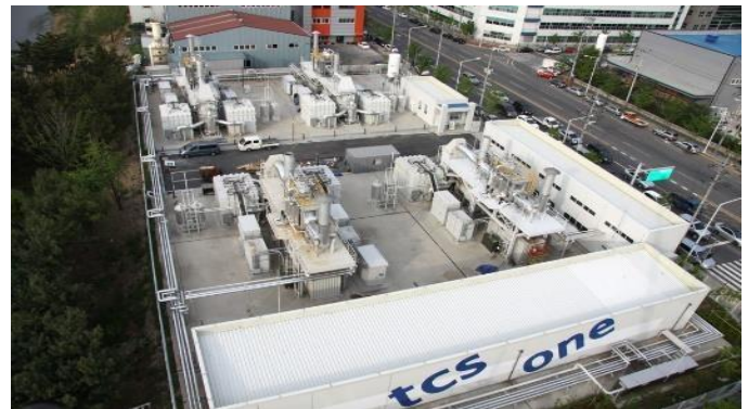
Figure 1. TCS1 Fuel Cell Power Plant in Daegu, Korea
